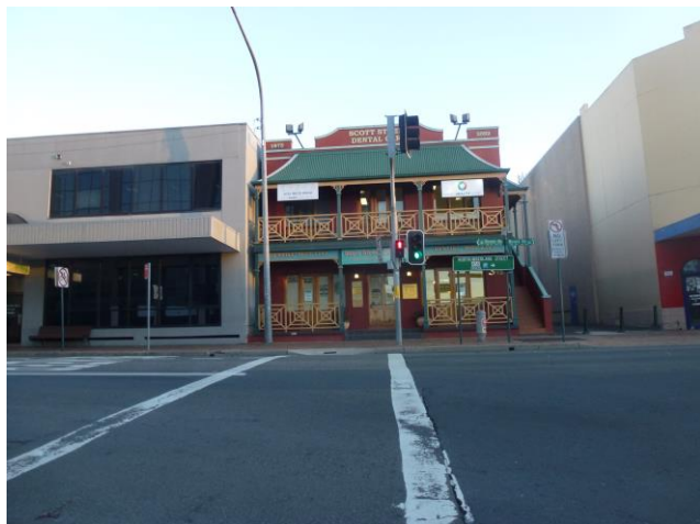
Figure 20: Two storey commercial building to the east of the George Street through site link
