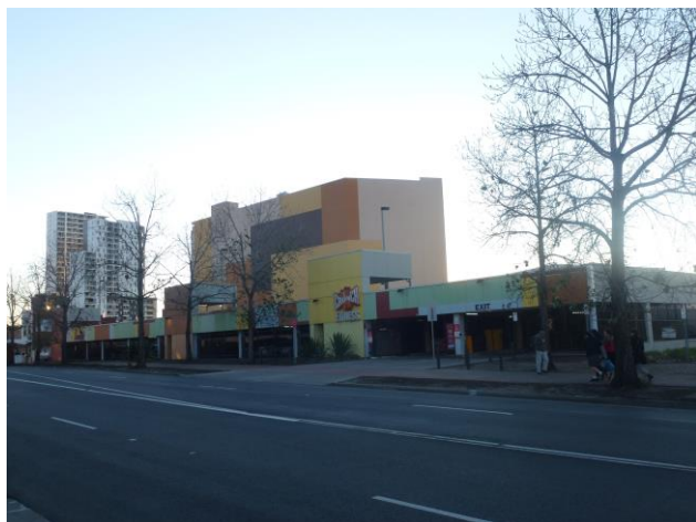
Figure 8: Above ground car parking structure as viewed from Terminus Street (south east)
