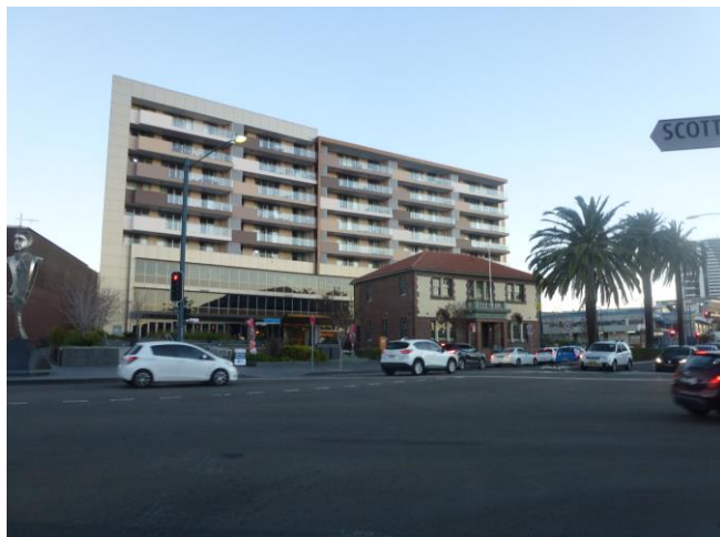
Figure 24: Nine storey mixed use residential building to the west
