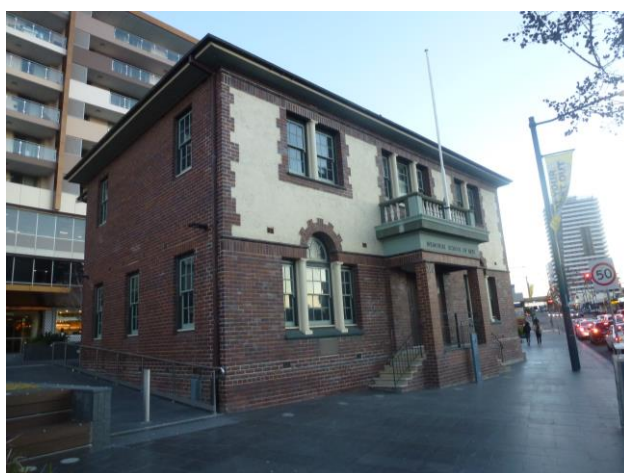
Figure 11: Memorial Arts Building
