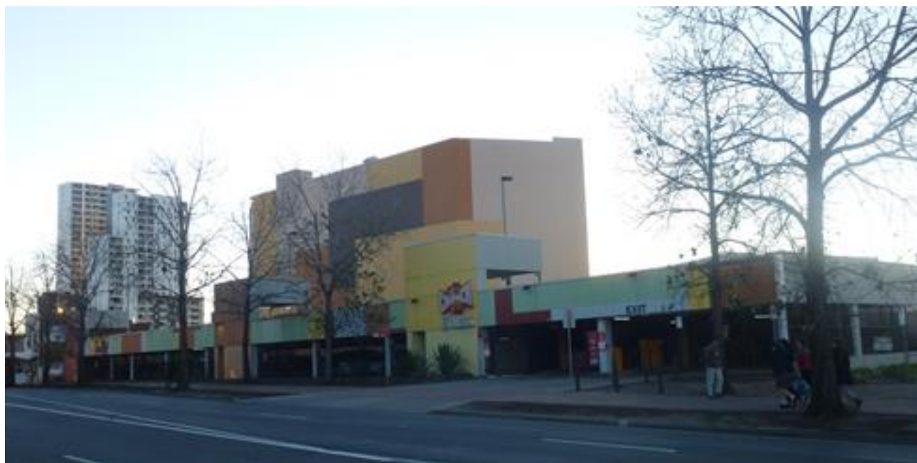
Figure 42: Rear Party wall of the mixed use building located at 300 Macquarie Street
