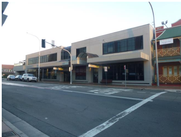
Figure 21: Two storey commercial building at the intersection of Scott and Terminus Street
