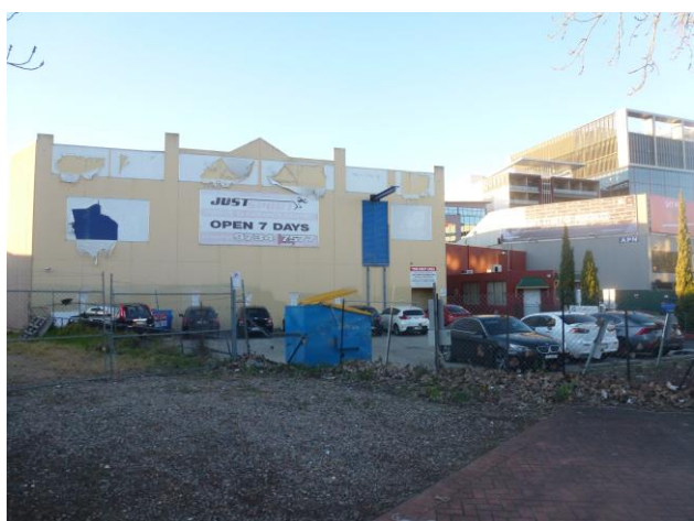
Figure 10: Rear car park of the commercial building as viewed from Terminus Street (south east)
