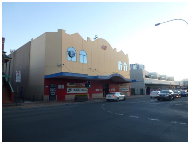
Figure 9: Commercial building occupying the site as viewed from Scott Street (north east)
