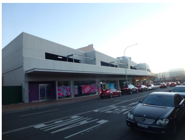
Figure 6: Commercial building occupying the site as viewed from Scott Street (north east)
